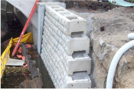
To strengthen the walls foundation and its ability to resist washout, rebar dowels were placed into the concrete foundation, which extended through the centre of each Verti-Block on the first course. The first course of Verti-Blocks was then filled with concrete to anchor them to the concrete foundation. For additional durability, the wall was reinforced with geogrid, which was laid between each subsequent block course.
