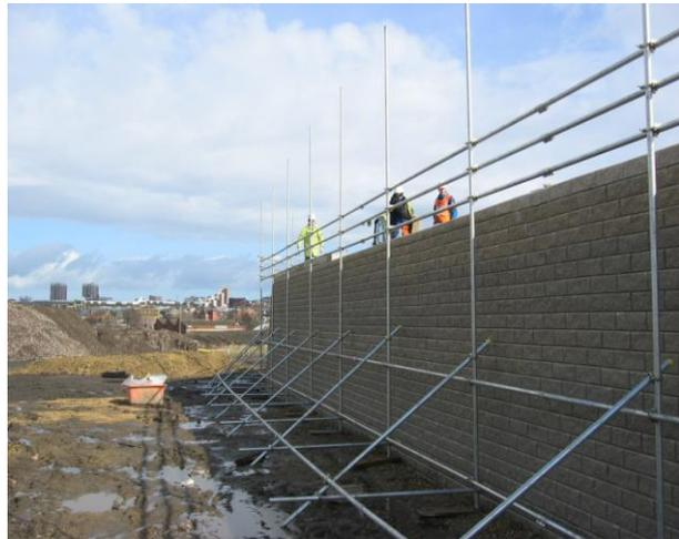
In some situations, such as when building adjacent to rivers and railway lines, there may be insufficient space in front of the wall face to accommodate a conventional scaffold frame.
