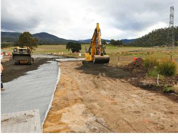
Due to the buried pipelines, we were restricted from excavating to the desired depth for 'sound' subgrade and pavement thickness. The geogrid provided protection of the excavated subgrade and good interlocking properties for the granular material. This resulted in less pavement thickness required for the road.
