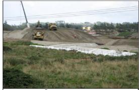
Use of bidim<sup>®</sup> for drains and sediment ponds
