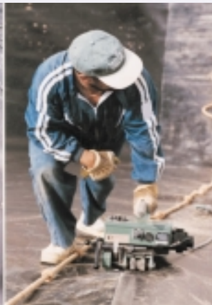
Automatic welding with hot air or wedge
