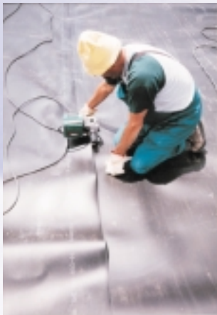
Automatic welding with hot air or wedge
