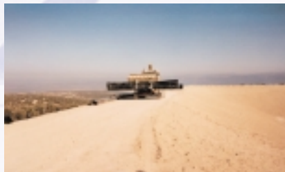
Panel cutting and transport : Platform minimum 3,5 m width
