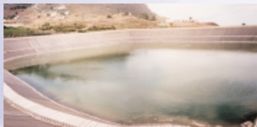
Ballasting with intermediate berm
