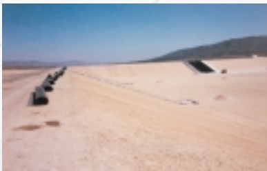
Distribution of cut panels at the crest of the slope
