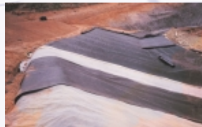
Excavation of anchorage ditch
