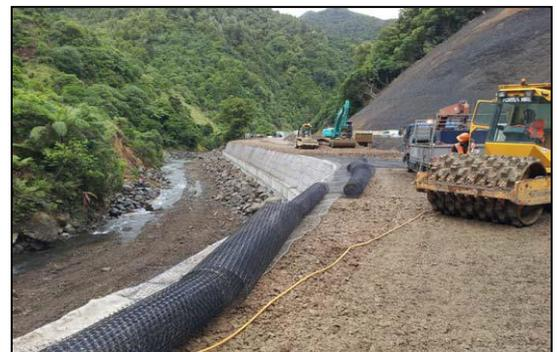
Tensar TriAx<sup>®</sup> is installed in preparation of the pavement
