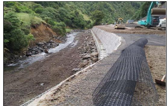
Tensar TriAx<sup>®</sup> laid over Green Terramesh wall
