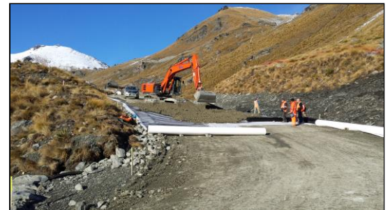
Laying bidim® and Tensar TriAx®
