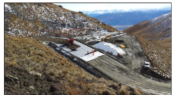
Aerial view of the bidim® and TriAx® installation
