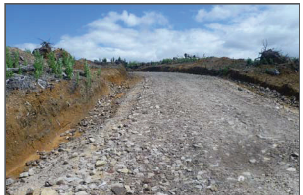
TriAx installed under this forestry access road
