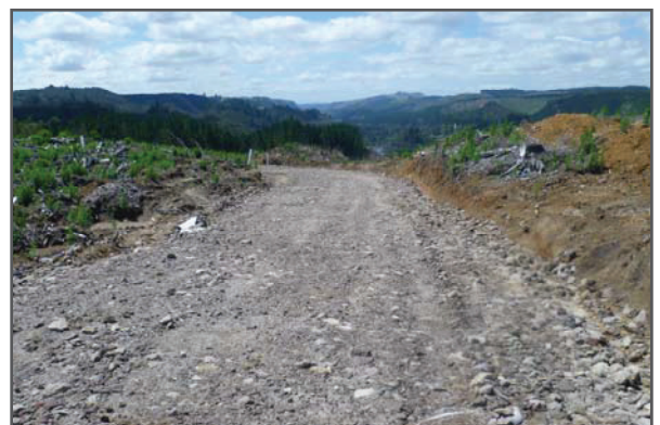
The access road after completion of the timber extraction
