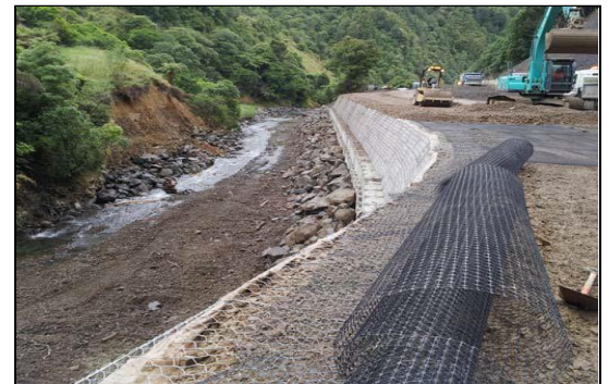
Tensor TriAx ® laid over Green Terramesh wall
