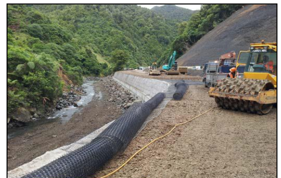
Tensor TriAx ® is installed in preparation of the pavement
