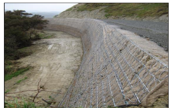
Green Terramesh wall
