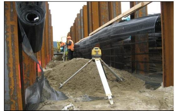
Tensor RE wrap around construction between H Piles
