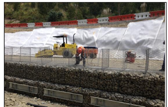
Installation of gabions
