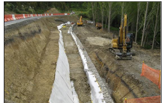
Preparation and work in progress
