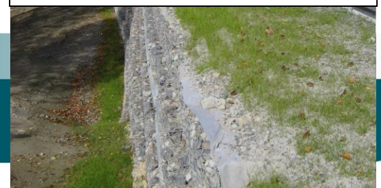
Completed Terramesh Wall in use
