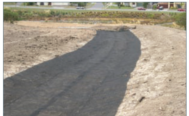
Finished placement of Enkamat
