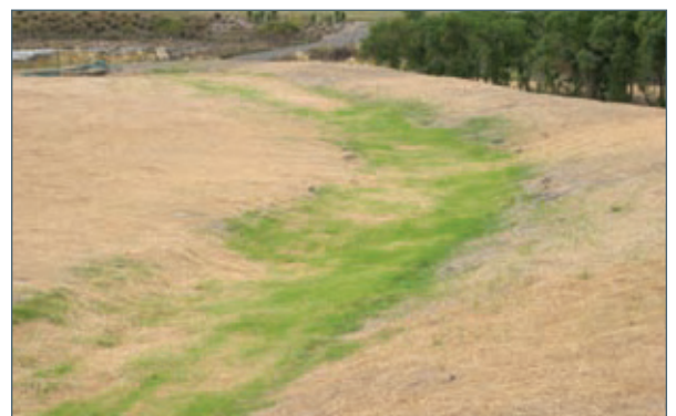
Enkamat & Biomac lined spillway with grass now striking
