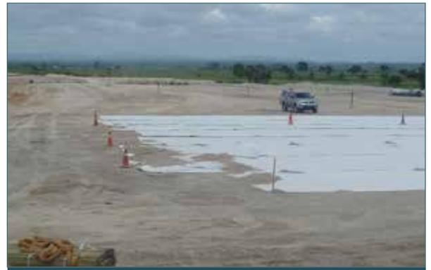
Mirafi installed installation during embankment
