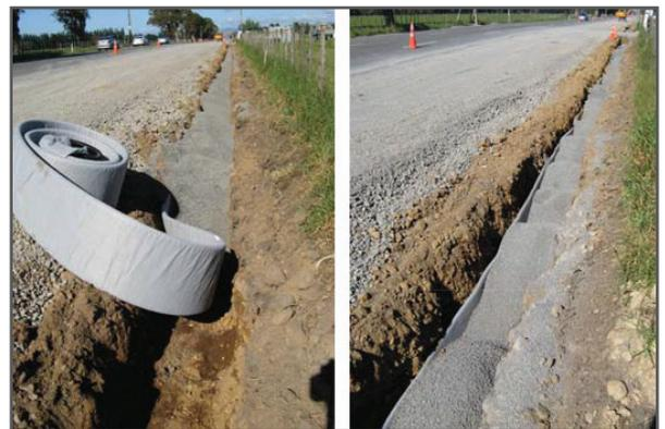
Laying of Megaflo on the edge of the trench
