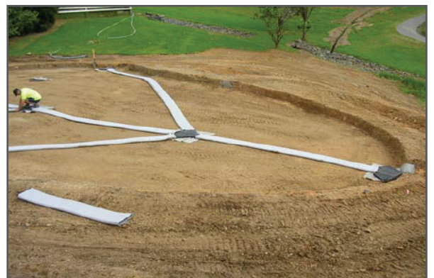
Placing Megaflo® onto the prepared profile
