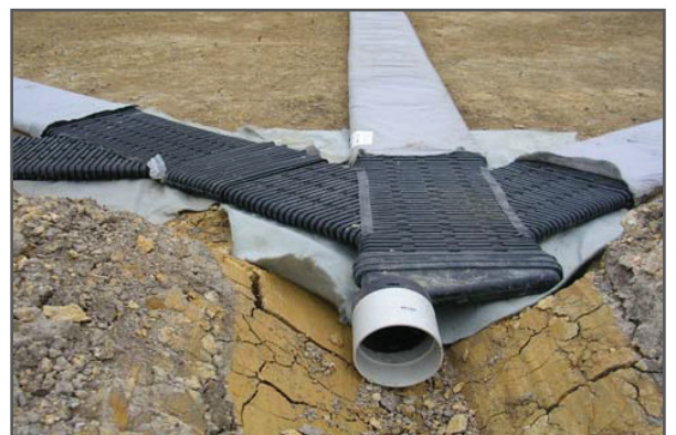
Installing Megaflo® with Dual Herringbone Fittings
