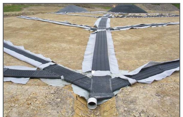
Megaflo® 300 with bidim® geotextile sliced open
