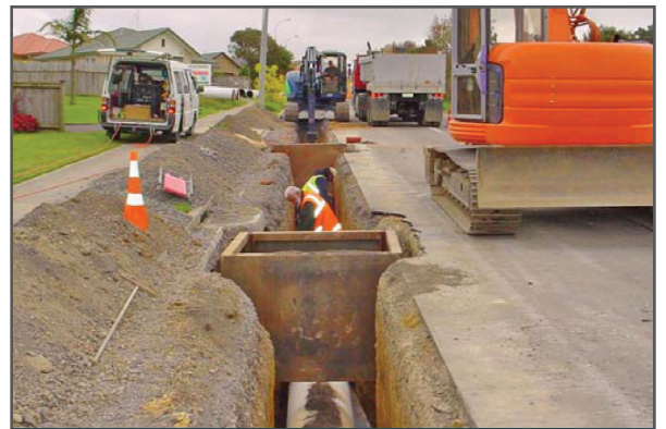
2.3m deep trench with mains pipe
