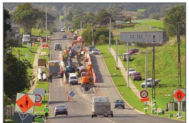
Construction along Alfriston Rd
