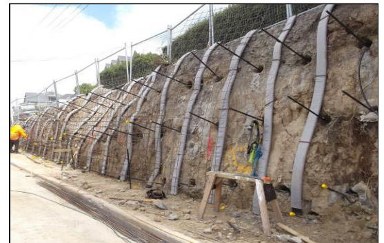
Laying of the Megaflo® drainage
