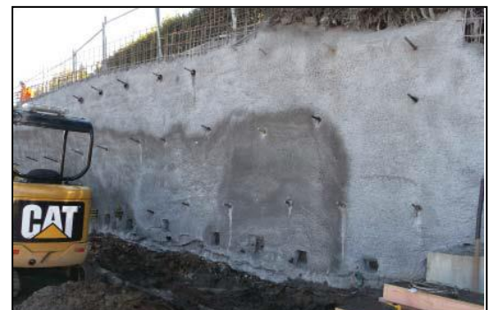
Shotcrete walls over the Megaflo®
