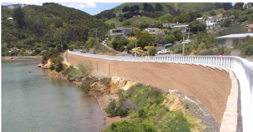
Completed Keystone TW3 Wall
