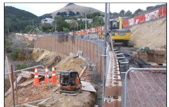
Keystone TW3 wall construction
