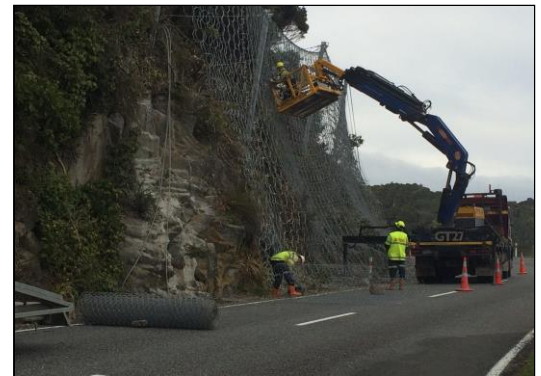
Installation of intercepting panels
