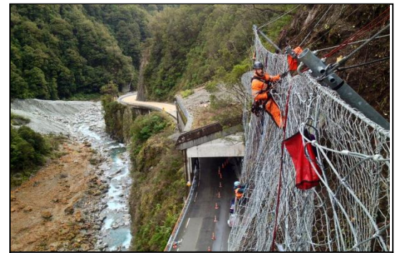
Completed rockfall hybrid fence (Photo courtesy of Abseil Access Ltd)
