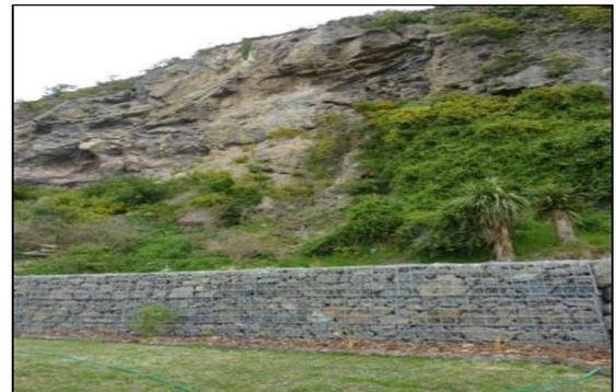
Completed GTM embankment with rockfall face
