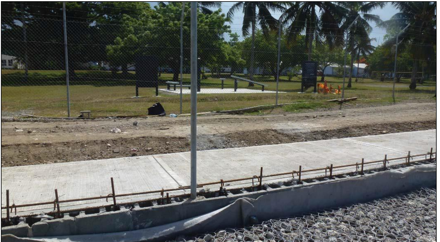
Construction and completion of Gabion and Reno mattress wall
