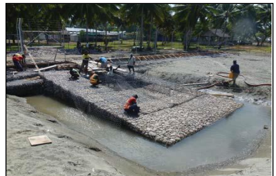
Construction of boat ramp
