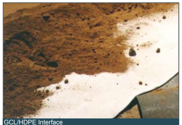
Fill placement over ELCOSEAL
