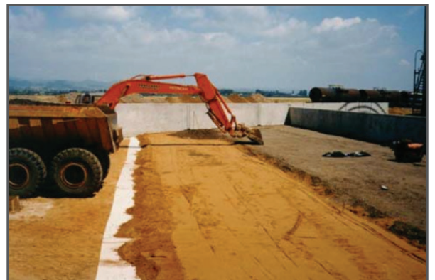
Fill placement over ELCOSEAL
