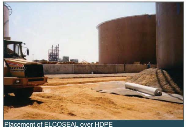
Placement of ELCOSEAL over HDPE
