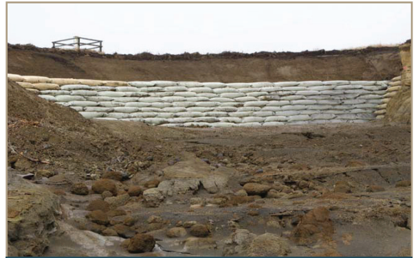
Completed section prior to erosion mat placement
