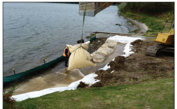
ELCOROCK® containers being placed
