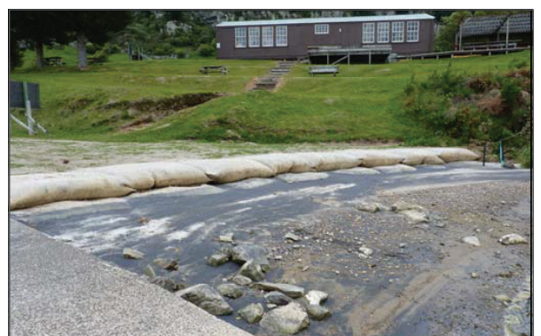
Finished project with ELCOROCK®
