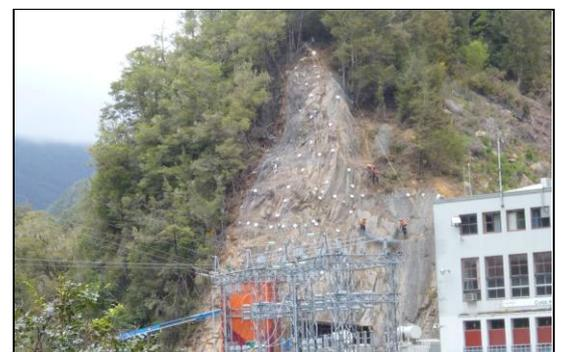
Steelgrid® HR30 mesh protecting the switchyard
