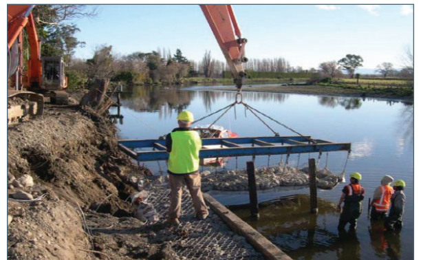
Installation of Reno mattresses
