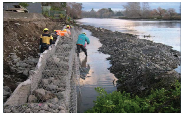
Gabion installation in process
