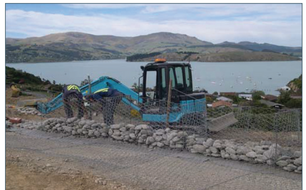
Terramesh Walls Construction
