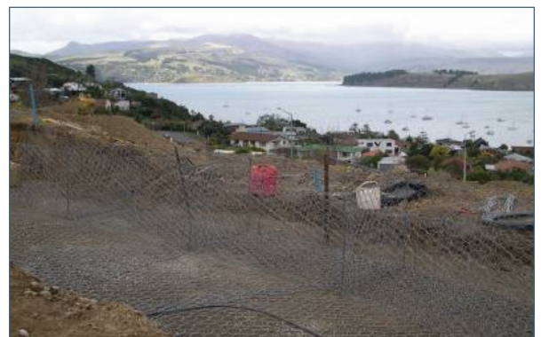
Terramesh System with gabion facing
