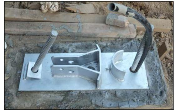
Base plate on concrete plinth footing
