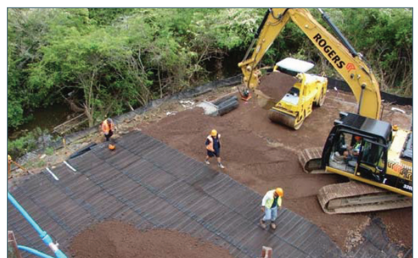
Placement of geogrid & fill
