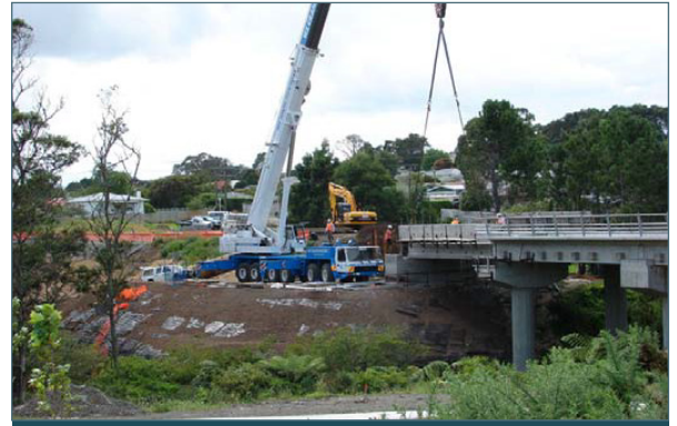
300T crane operation
