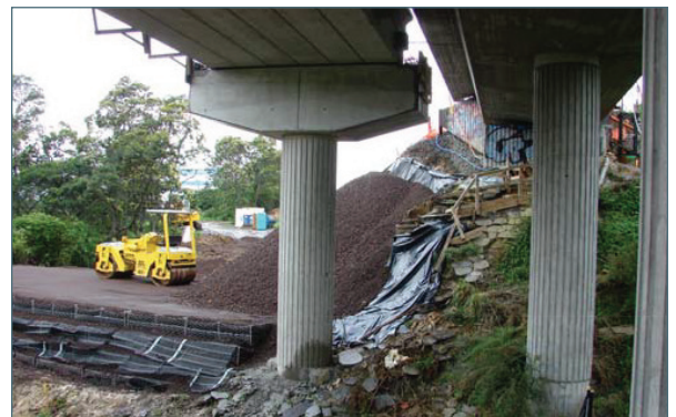
Lower prefilled gabion section
