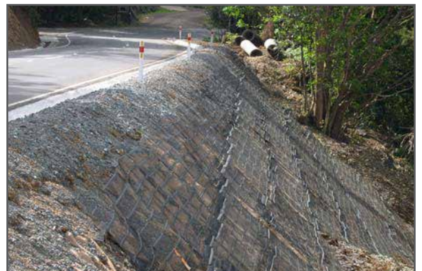
Laying Bidim, Biomac and Tensar
