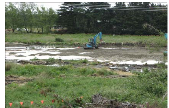
Installation of Mirafi PET
