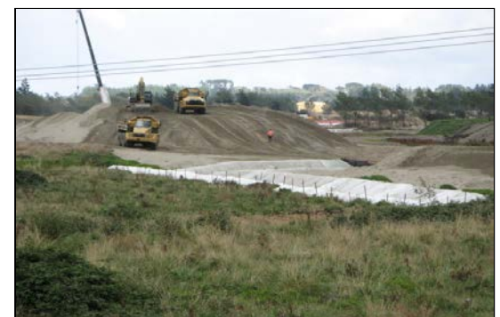
Use of bidim ® for drains and sediment ponds
