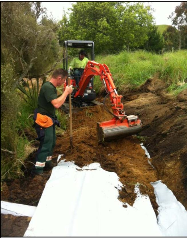
Installed bidim® geotextile as a separation layer
