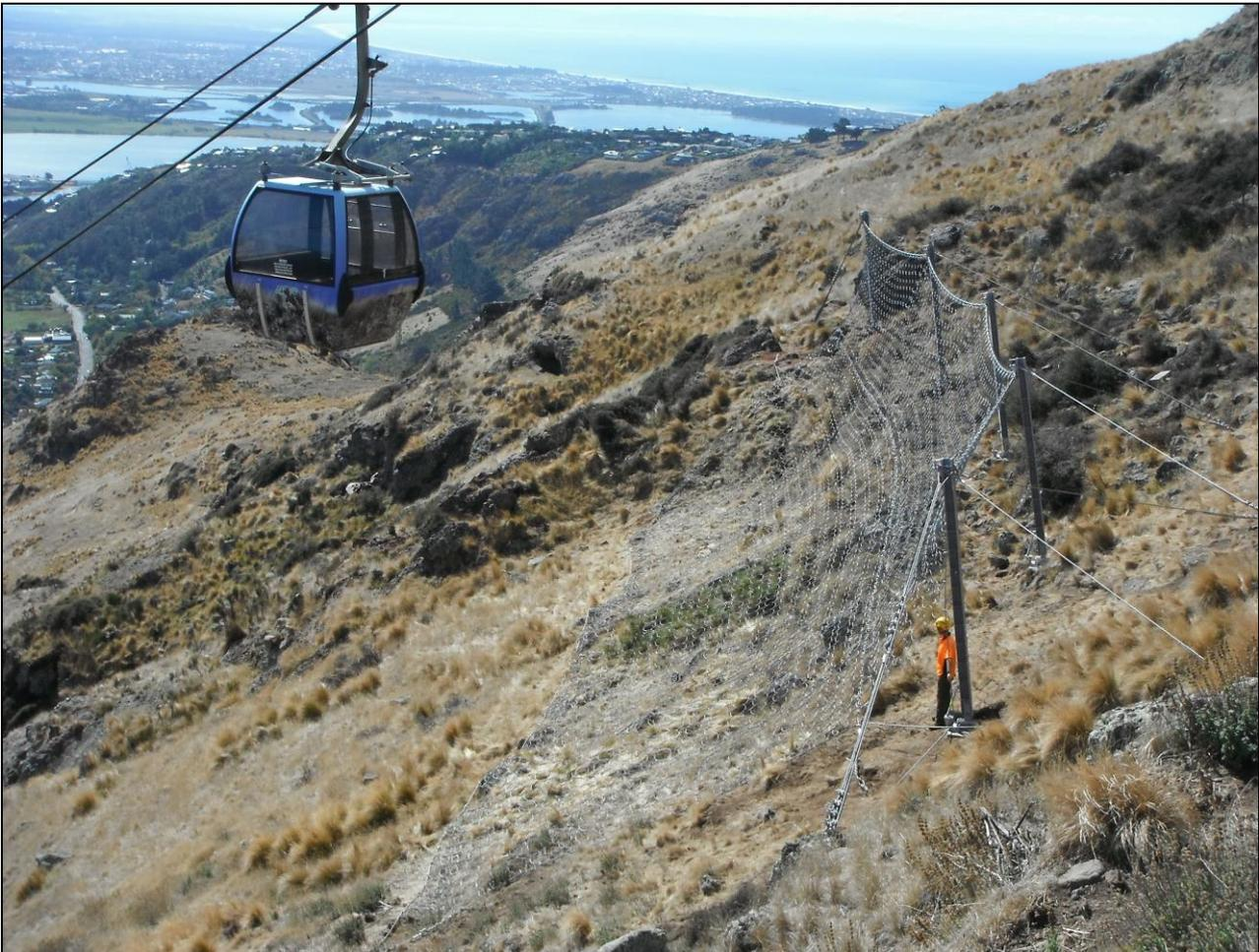
Completed Attenuator Fence Photo courtesy of Solutions2Access Ltd
