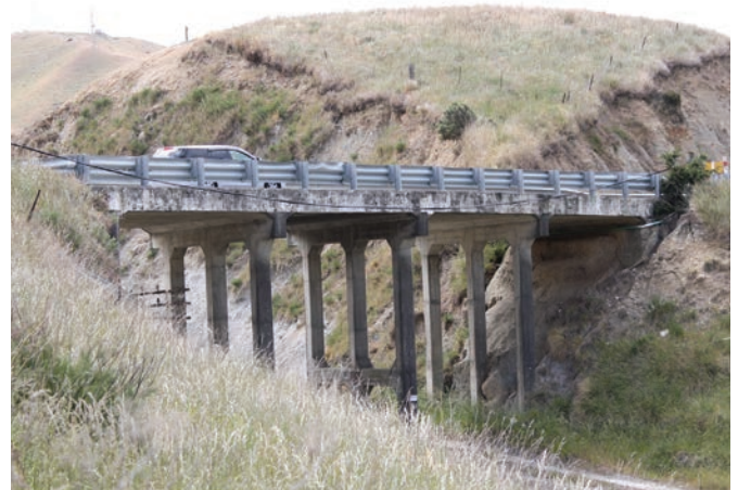
EXISTING BRIDGE AND NORTHERN END
