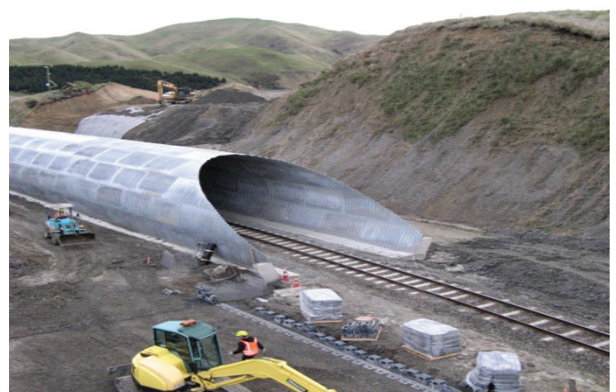
CONCRETE FOUNDATION FOR KEYSTONE TW3
