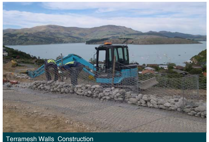
Terramesh Walls Construction
