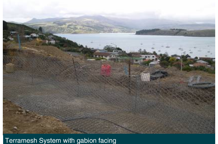
Terramesh System with gabion facing
