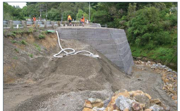
Construction of Green Terramesh structure
