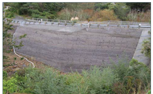
Completed Green Terramesh structure at Bryants Bridge
