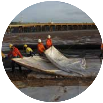
Mirafi® PET High Strength Woven Geotextile
