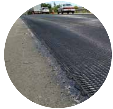
GlasGrid® Pavement Reinforcement Geogrid
