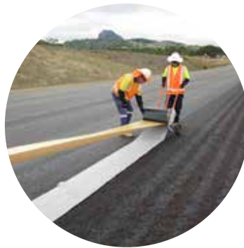
Bitac® Multi-Laminate Asphalt Reinforcement Tape
