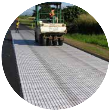
Tensar® ARG Asphalt Reinforcement Grid
