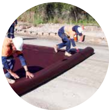
Mirafi® RSi High Strength Woven Geotextile
