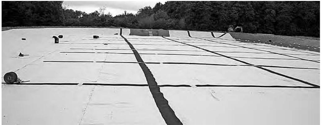
**Figure 6 - Grid layout of the basin surface by strips of 1m every 10 linear meters minimum**
