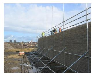
In some situations, such as when building adjacent to rivers and railway lines, there may be insufficient space in front of the wall face to accommodate a conventional scaffold frame. This has been overcome by two methods: i) fixing rawl bolt eye rings into the block face at appropriate centres to accommodate the
