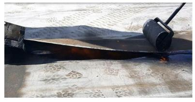
testing, visual and air lance testing of every seam, and trowelling of the molten material at welding.
