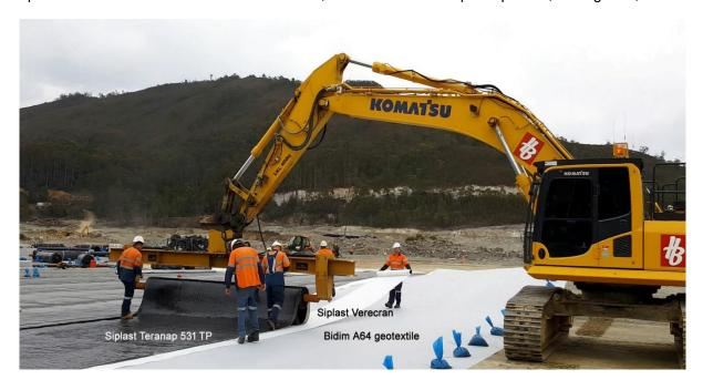
accurately place the liner with a 200mm overlap. This enabled Aeramix to install over 6,000m<sup>2</sup> per day, when conditions allowed. As the liner was being placed over Bidim A64 geotextile, a
