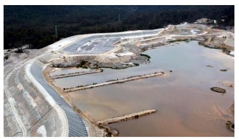
Hazell Brothers drilled, blasted, excavated, crushed, and moved over 1 million cubic metres of material during the construction, and Geotas installed 190,000m² net area of the Teranap 531 liner and 250,000m² of upper and lower cushioning geotextile.
