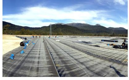
grout curtain. The scope in general terms, was to install approximately 2kms of cement / bentonite slurry in a deep trench around the perimeter of the existing dam, to create a waterproof seal down to bedrock. The Teranap Bituminous liner was then anchored into the cut-off wall, and laid over the surface where crushed material was used to construct the new dam walls. The liner was then installed up the face of the new walls, and secured in an anchor trench.
