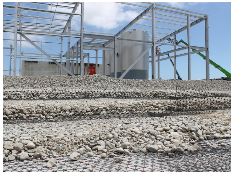
Close up of Tensor TriAx layers.
