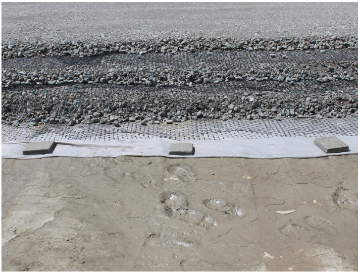
Illustrates soft subgrade.
