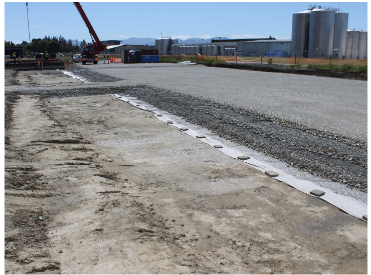
Site prep and first section install.
