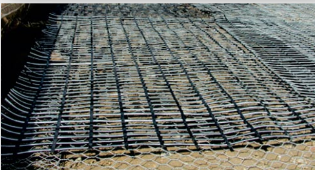
Terramesh Green or System units acting as secondary reinforcement and permanent shuttering
