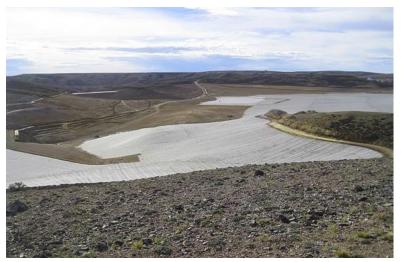
The solution is collected and guided to the basin. This recovery process requires a perfect waterproofing system in order to avoid widespread soil contamination. The bituminous geomembranes Teranap TP 531 and 431 have met the most rigorous requirements of the project.
