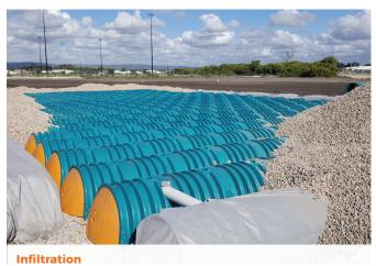
A large ecoAID stormwater collection tank used for infiltration.
