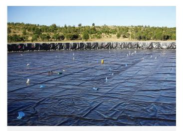
**INSTALLATION OF THE PRIMARY LINER** The primary liner was installed in large prefabricated panels which were lifted over the tank walls and placed in position.
