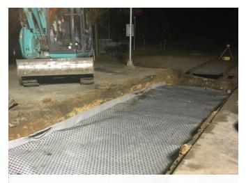
PLACEMENT OF GEOSYNTHETICS Tracktex and Tensar TriAx 190L rolled out onto the clay subgrade
