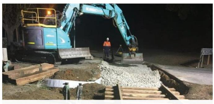
**REINSTATEMENT** The track formation is reinstated over the Tracktex and Tensar TriAx 190L layers
