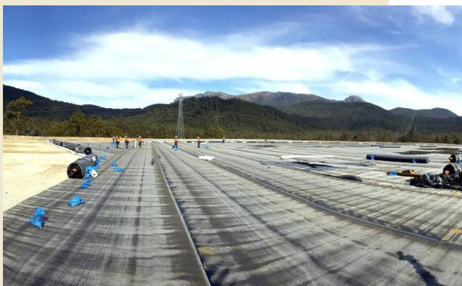
Teranap was chosen for this project for its weldability and flexibility to conform to irregular shapes and surface conditions.
