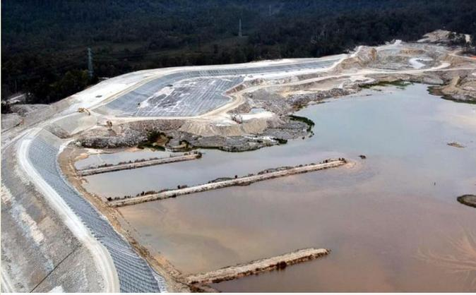
Geotas installed 190,000 m<sup>2</sup> net area of the Teranap 531 liner and 250,000 m<sup>2</sup> of upper and lower bidim cushioning geotextile.
