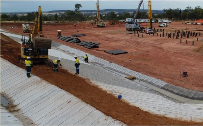
Concrete Canvas was the best option to fill the brief of both channel lining and erosion control.
