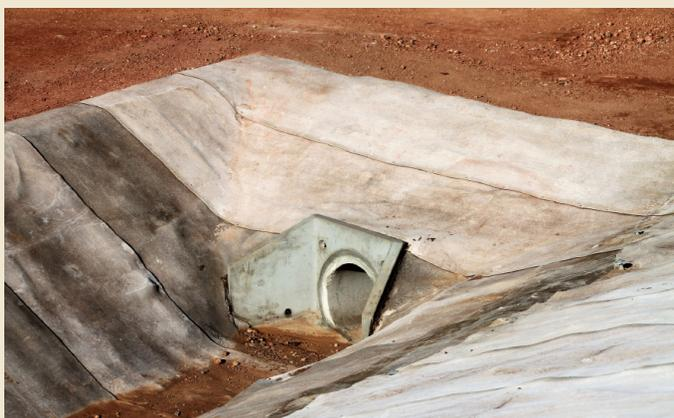
Concrete Canvas was laid transversely after the removal of vegetation on cut batters in drains.
