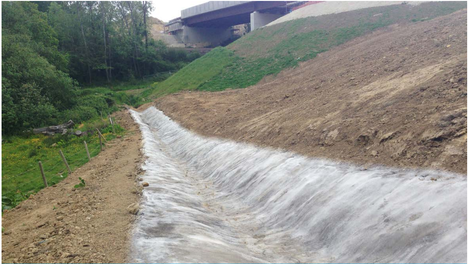
Immediately after installation
