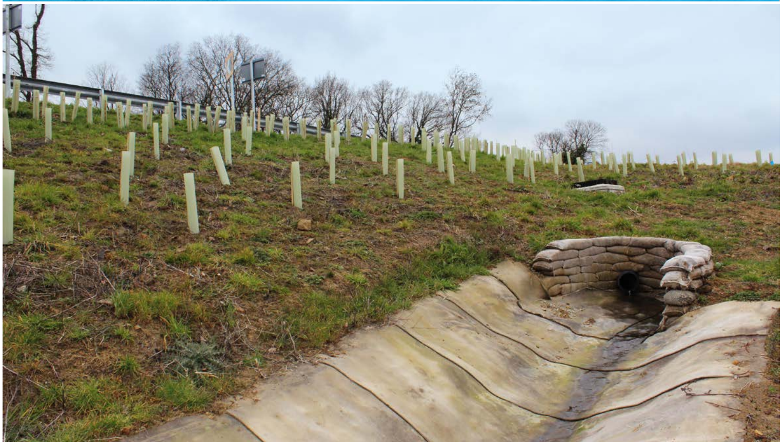
CC connected to concrete sandbag headwall
